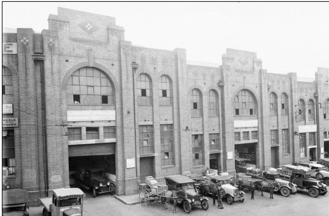
Figure 14: Quay and Valentine Streets; The Producers' Cooperative Distribution Society. SLNSW Home and Away - 35022
