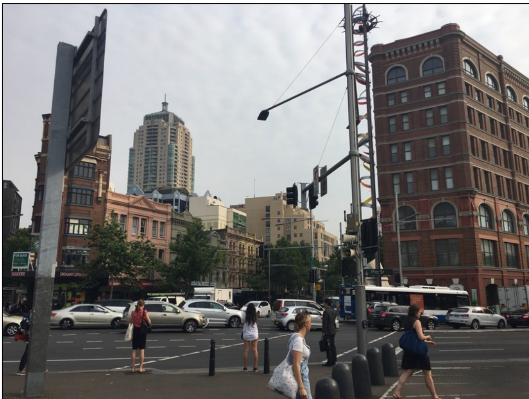
Figure 19: The Former Commercial Building, 'Orchards Chambers at the intersection of Pitt Street and Eddy Avenue.
