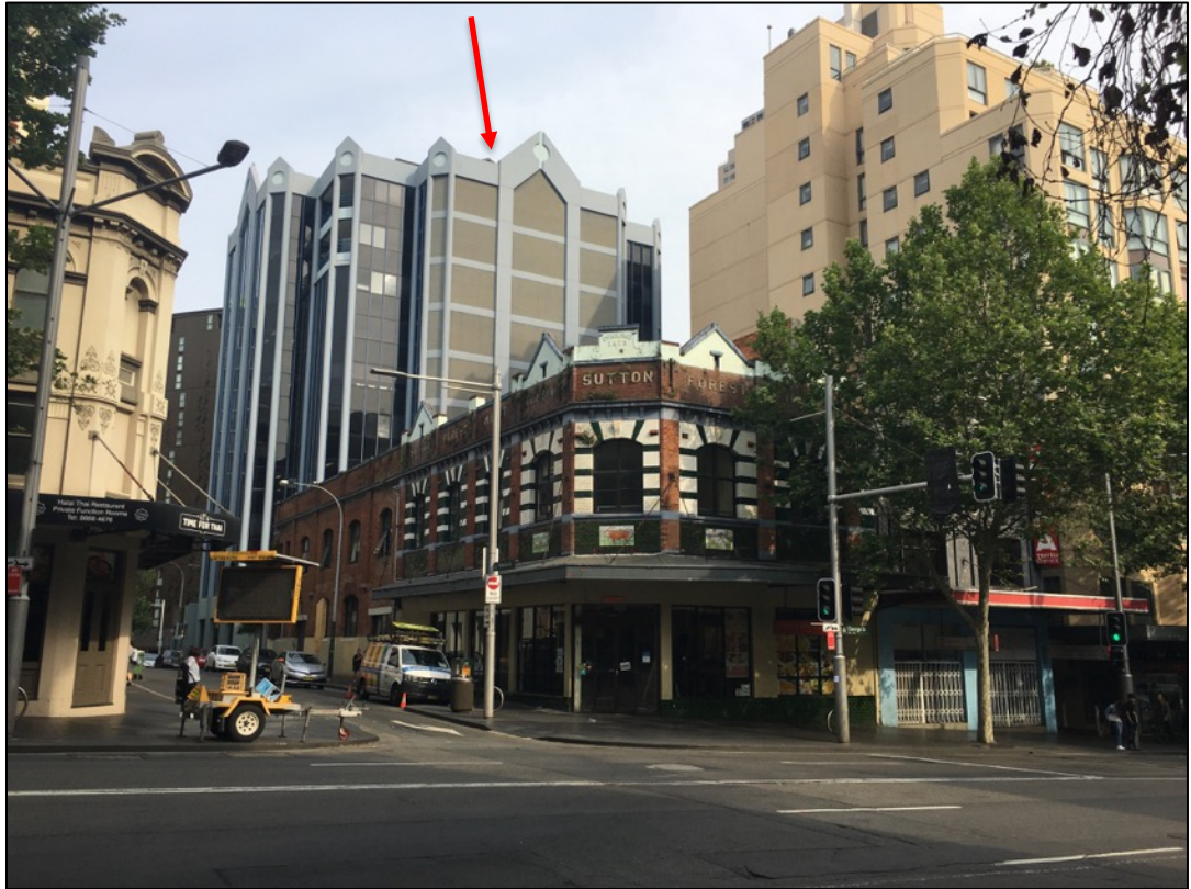
Figure 28: The site as viewed from George Street behind the former Sutton Forest Meat building.
